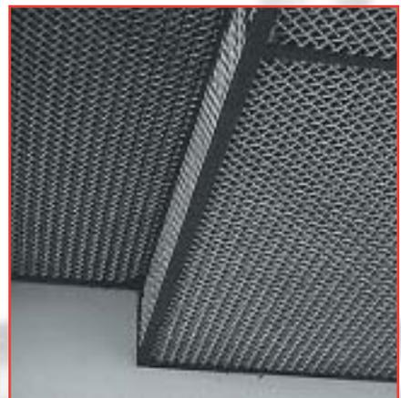
*Soffit Detail; Woven Wire Mesh*
